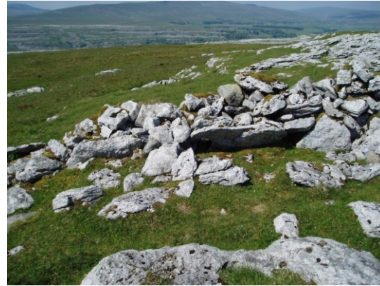
Fig.7 Detail of the wall showing how parts of it were constructed, with long thin slabs set on both sides and stone in between
