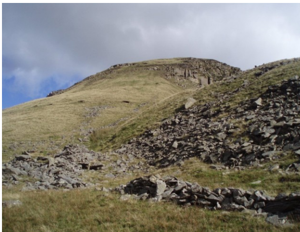
Fig.8 The gritstone wall (ING 116) descending the flank of Ingleborough by Fall's Foot
